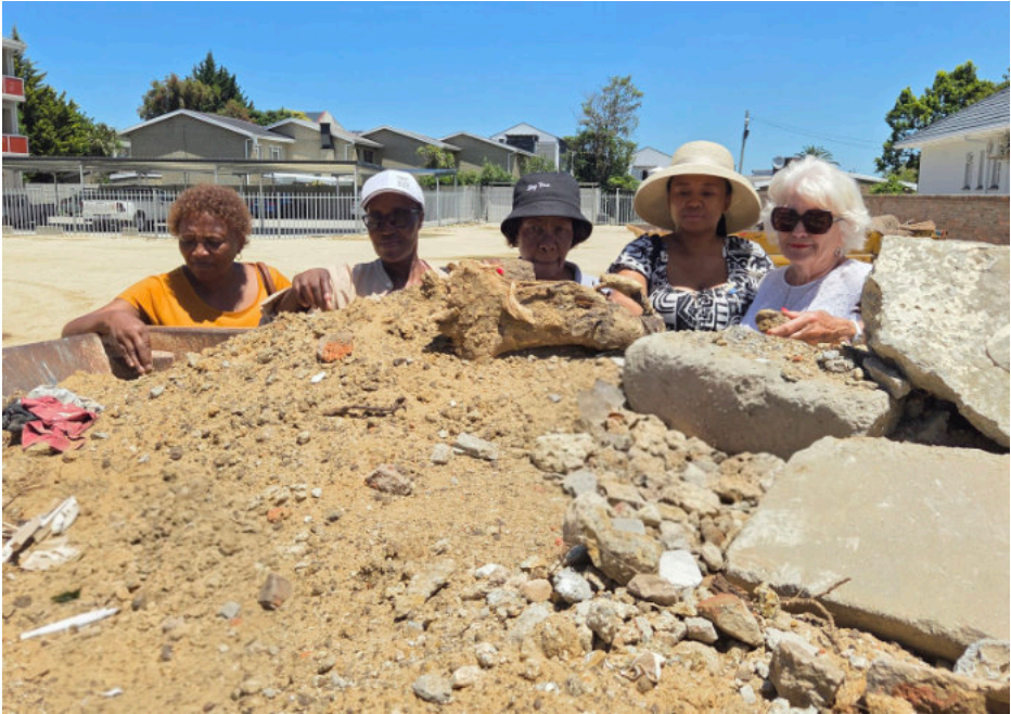
Members of the Maloti and George clubs visit the site of the May 2024 building collapse, where survivor Shadrack Maine had worked.
